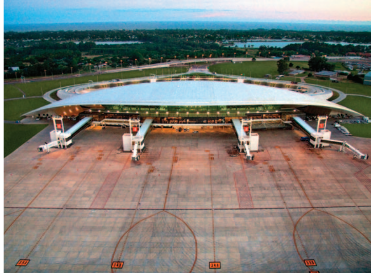
Landing track of the Carrasco International Airport, Montevideo, Uruguay
